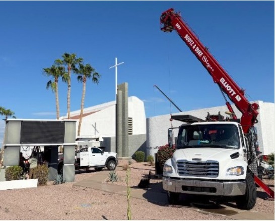
September 15, 2026 - New panels installed
